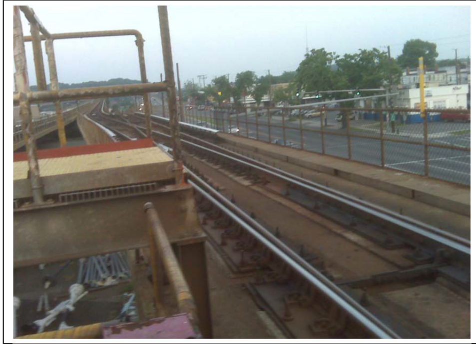
Picture 4 - D & G Platform, Track 1
