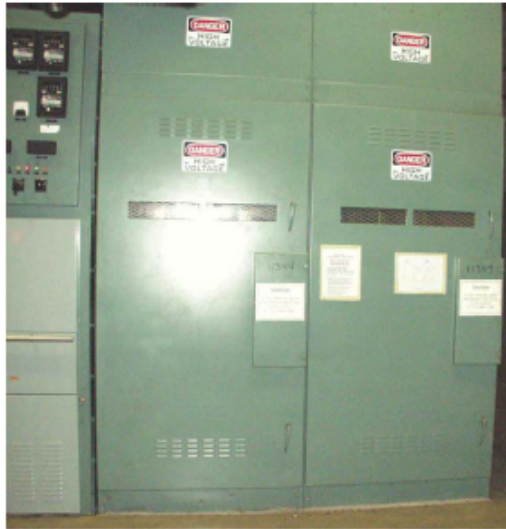
Fig. 1 WESTINGHOUSE 34.5KV LOAD INTERRUPTER SWITCH TYPE WLI
